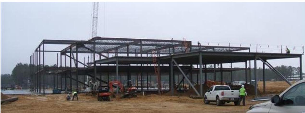
View from Rear of C2F
